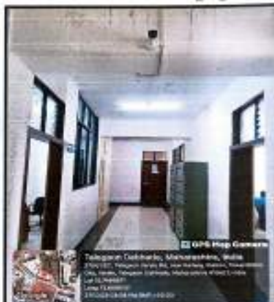
Camera in Corridor
