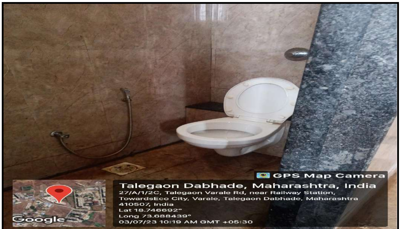
Disable Friendly Washroom
