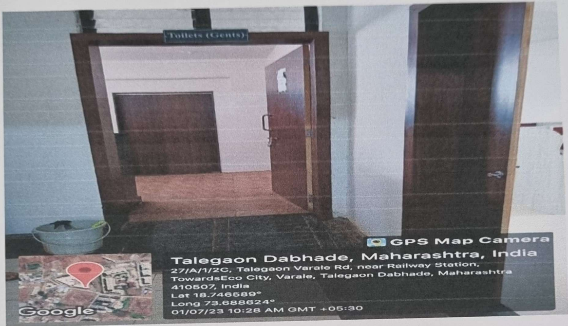
Ramp at the Toilet
