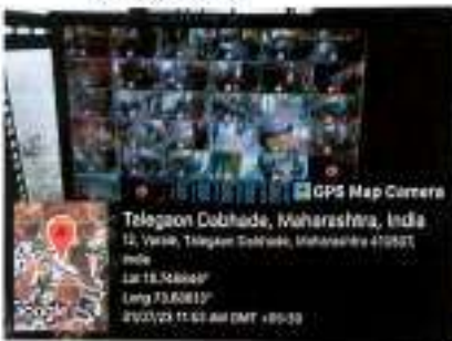
CCTV Access at Server Room
